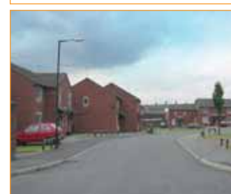
Modern Residential: turns its back on the surrounding area. Character is not distinctive - could be anywhere.
