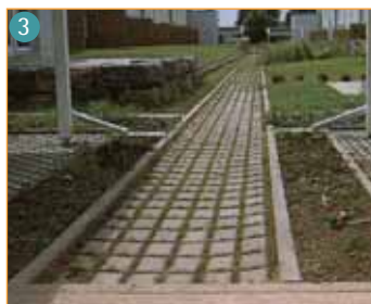
3 Drainage solutions should be integrated into the layout from the earliest stage. SUDS features can take many forms, and work with both urban and rural developments.
