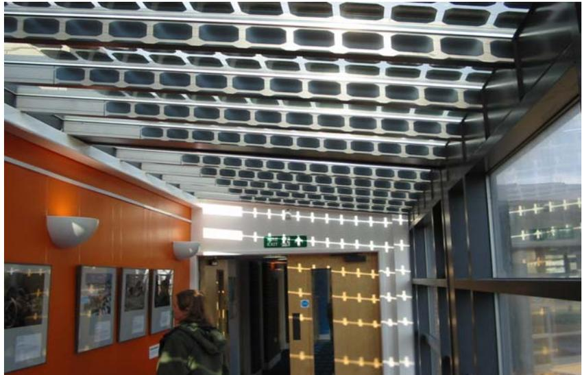
PV is also an ideal material that can be incorporated directly into roof tile, or glazing to act as a shading material (see photo 3) thus the cost can in part be offset by the use of expensive cladding or glazing materials at the design stage.
